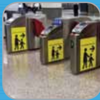
Access Control & Security
